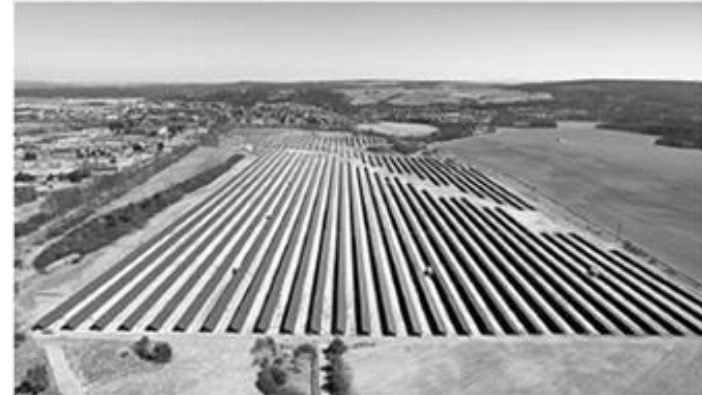
The free-field solar plant at Střebro in the Czech Republic (Courtesy: S.A.G Solarstrom AG).
