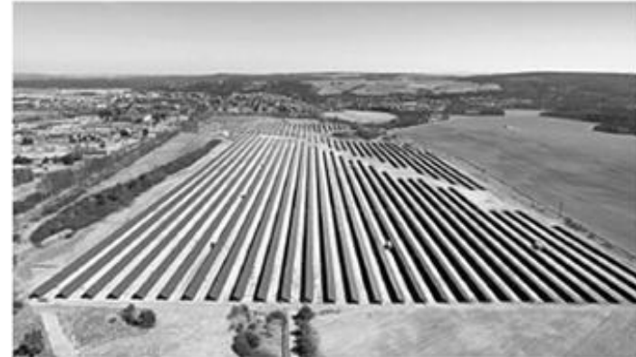
The free-field solar plant at Střebro in the Czech Republic (Courtesy: S.A.G Solarstrom AG).
