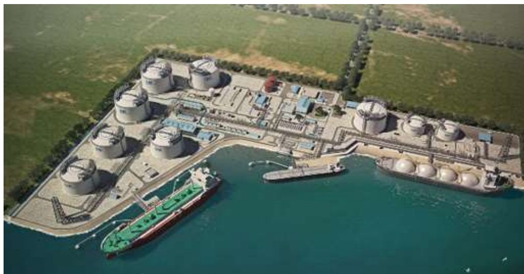
Figure 37 – Singapore LNG with extra tanks for trading
