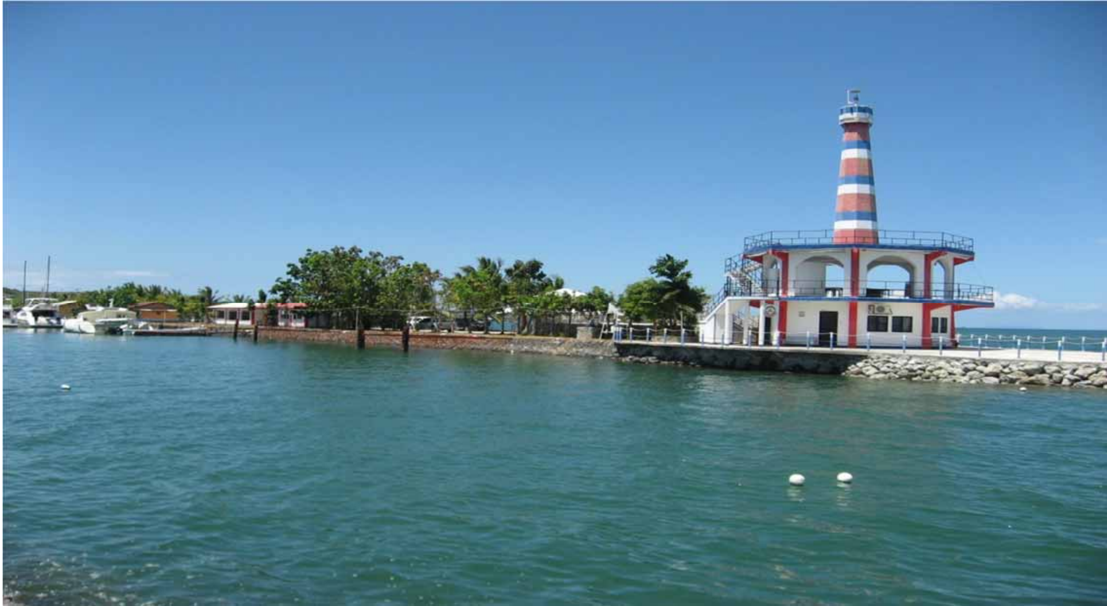
OLP No. 10 Light House, Dry Dock, and Shipyard L'Nor Marine Services, Inc. Liloan, Cebu
