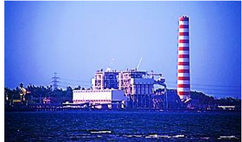
116-MW BUNKER FIRED POWER PLANT (ONE SUBIC POWER GENERATION CORPORATION)
