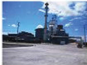
I-POWER- 2X12 MWe Biomass-Fired Power Plant
