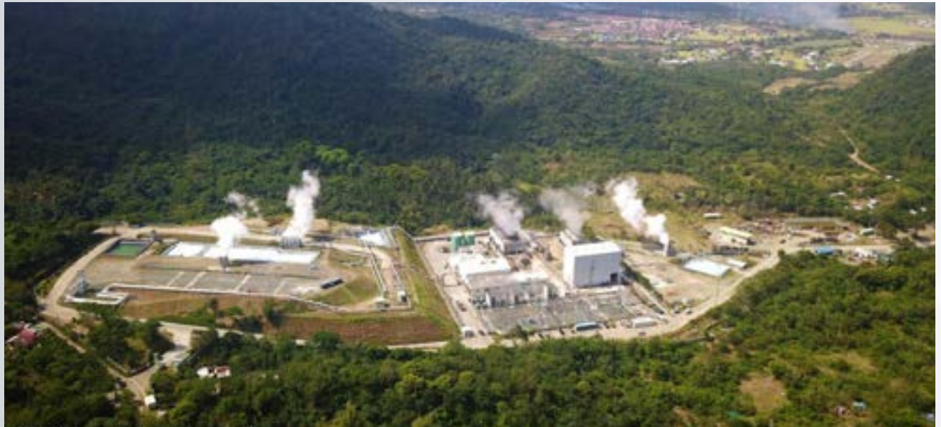
Figure 14. Maibarara Geothermal Power Facility in Sto. Tomas, Batangas
