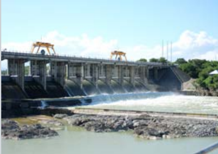
Figure 17. National Irrigation Administration- Magat River Integrated Irrigation System (NIA - MARIIS) Re-regulating Dam in Alfonso Lista, Ifugao / Ramon, Isabela
