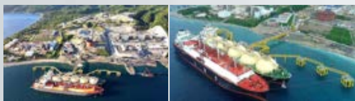
Figure 38. Linseed Field Corporation’s PHLNG Import and Regasification Terminal 2
