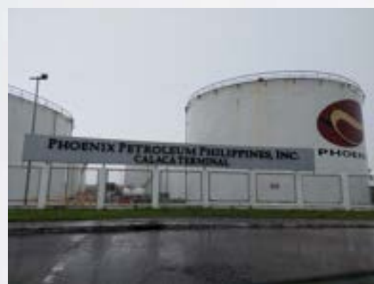
Figure 32. Liquid Petroleum Depot (Phoenix Petroleum’s Depot in Calaca, Batangas)
