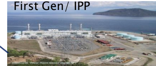
1,200 MW Ilijan Power Plant NPC IPP(KEPCO)
