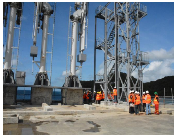
Regular Inspection & Monitoring of Natural Gas Facilities in the Philippines
